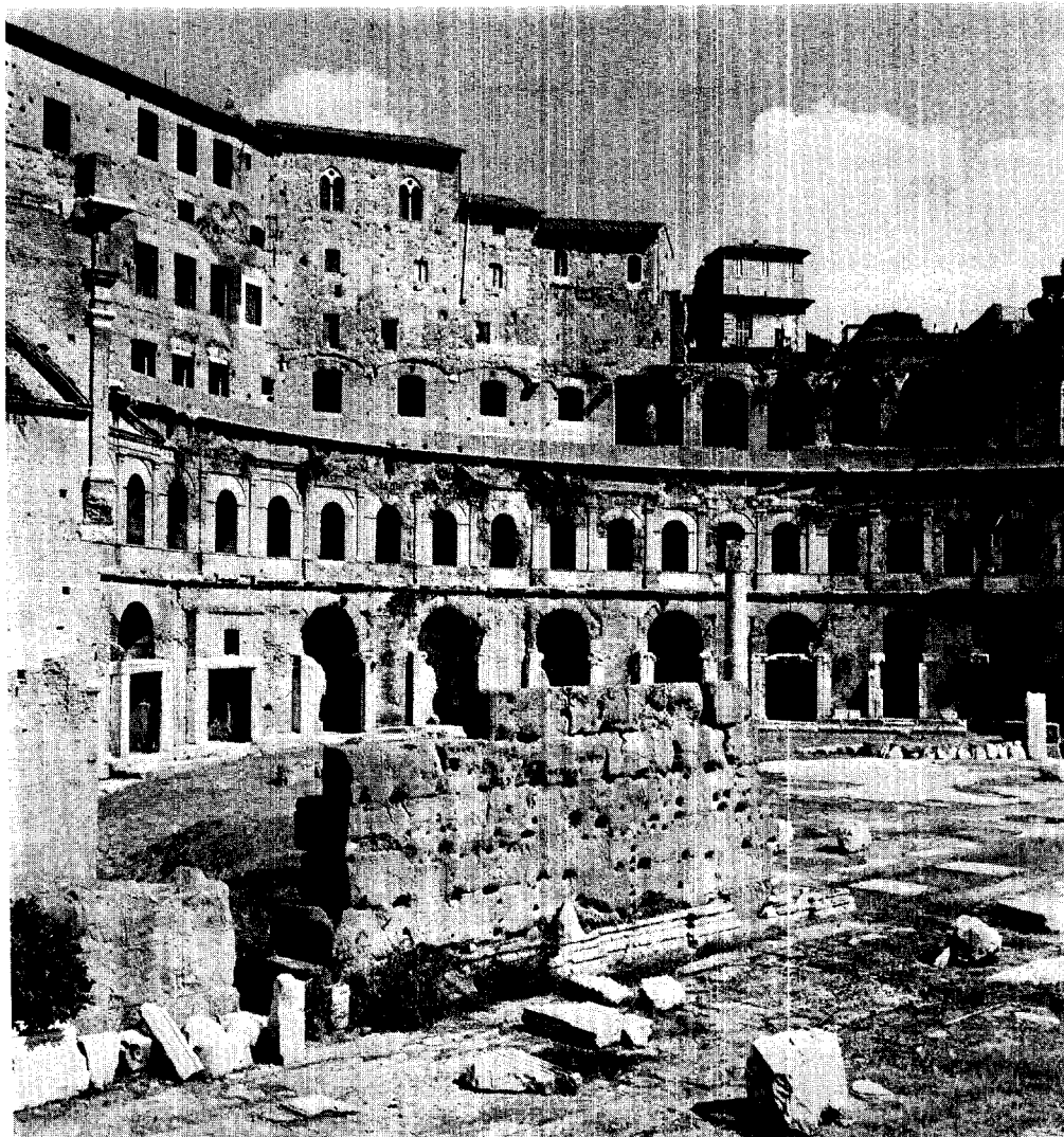
39.13 Trajan's Market (Mercatus). This market complex contained 150 shops ( tabernae ) and a two-storeyed hall. Streets at the back provided access to the building at three different levels.
