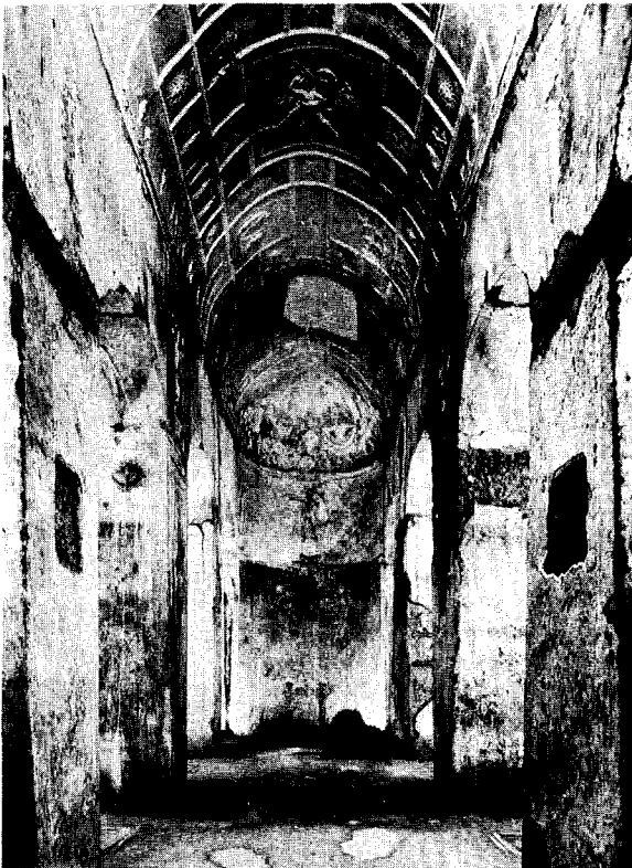
34.14 Subterranean basilica outside the Porta Maggiore at Rome. The rich stucco decorations depict mythological subjects; the hall may have been the meeting-place of a Neo-Pythagorean sect.
