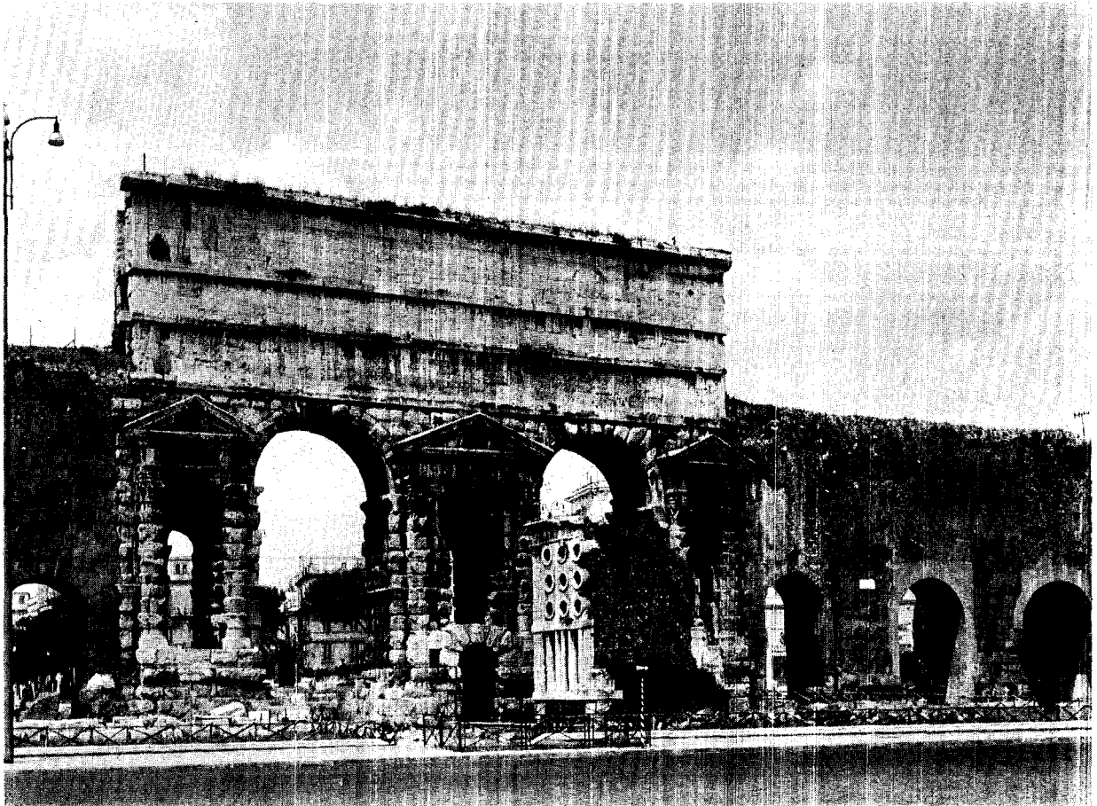
32.7 Porta Praenestina (Maggiore). These two monumental arches carried the Aqua Claudia and the Anio Novus over the Via Praenestina and the Via Labicana. They were incorporated by Aurelian into his city-wall as a fortified double gateway.
