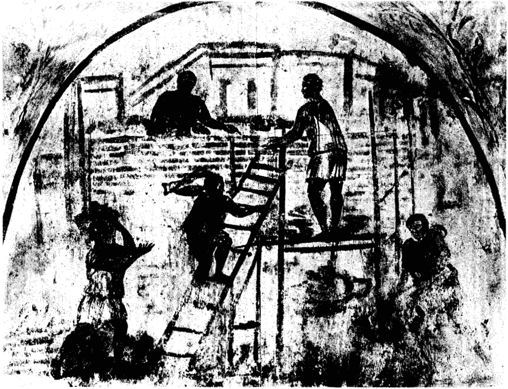
39.8 Wall-painting of building operations, from the tomb of Trebius Justus at Rome.
