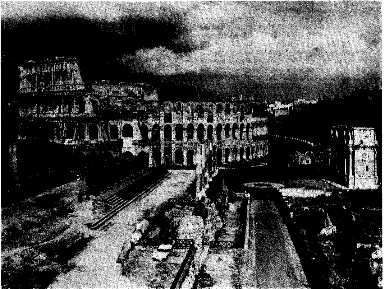
36.4 The Colosseum, with the temple of Venus and Rome in the foreground. The Amphitheatrum Flavium, generally known as the Colosseum, was begun by Vespasian and dedicated by Titus in A.D. 80. External view. It is elliptical and measures 180 metres long and 156 wide. It could contain an audience of some 45,000 to 50,000 spectators.
